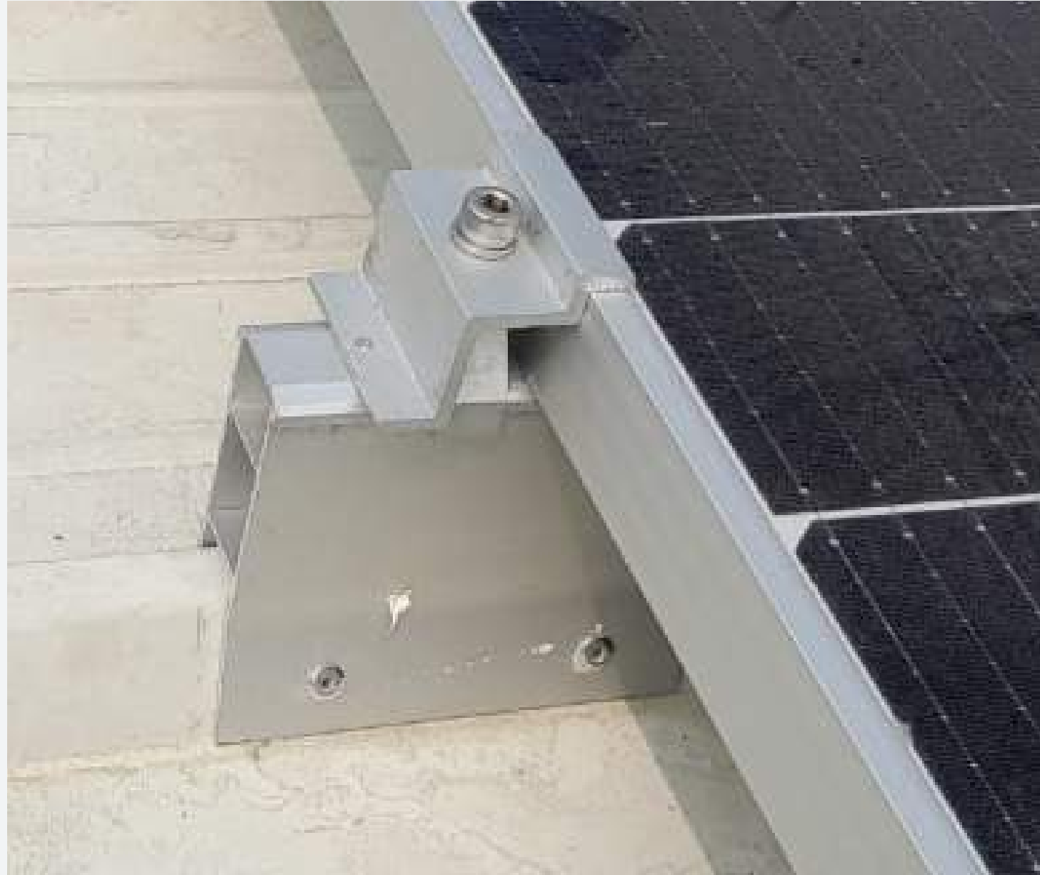
Fixing using rivets
