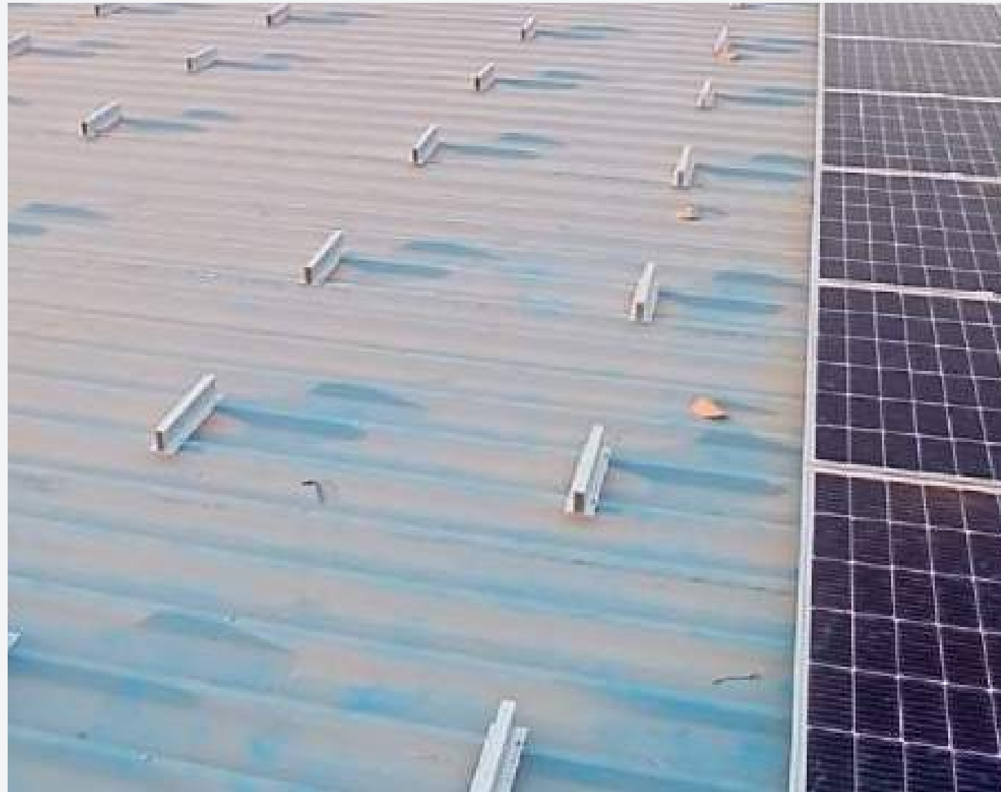
Fixing using rivets
